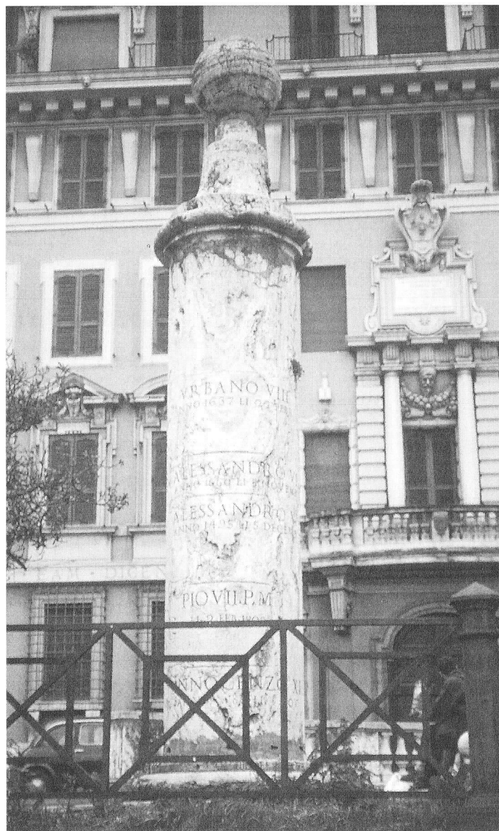
The Ripetta column is located in the Piazza del Porto di Ripetta, a former river port on the left bank of the Tiber, near the Ponte Cavour. The column was constructed by the architect Alessandro Specchi in 1704 to mark water levels during floods of 1495, 1537, and 1660 and is annotated with the names of popes during those flood years.
